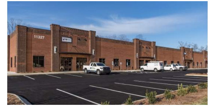
A new structure in Clear Creek Business Park offers space for multiple tenants.
